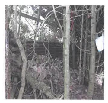
Inspection of the general road condition has revealed the dry-stone walls which retain the public road to be in poor condition and are subsiding into the site whilst damaging the roots of the hedge at the same time. This has forced the applicant to construct a steel and timber retaining wall to protect the land immediately adjoining Lindisfarne and runs parallel with the public road to the end of the rear garden.
