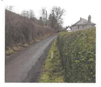
Bollards have been installed by the Council on the grass verge in recognition of the problem to protect the application site from road traffic driving over the defective dry-stone walls, further exacerbating the passing problems. The proposals detailed in this application will result in a new retaining structure to consolidate the road sub-structure and protect the hedge roots.
